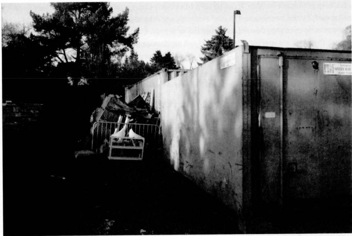
Purely utilitarian shipping contains and incongruous surface treatment.
